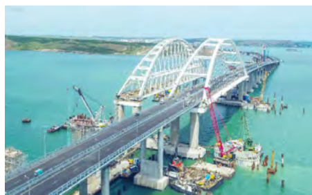
Figure 4: The Crimea Bridge under construction
