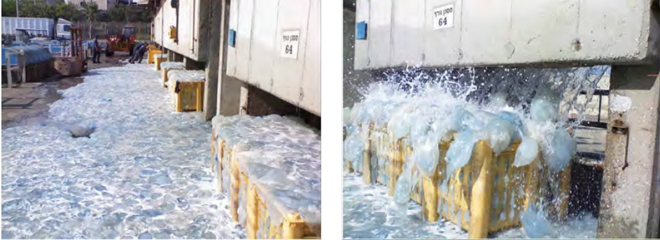
Figure 3: Jellyfish discharged from the filter of the Orot Rabin power station
