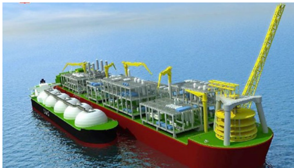
Figure 12.3 Facility for gas production and a facility for liquefaction and loading onto LNG tankers.
