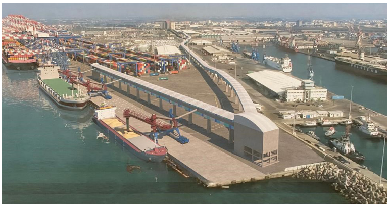
Figure 5: illustration of a pier that specializes in the conveyance of seeds to the Ashdod granaries, which will operate with an unloading capacity of up to 1,500 tons per hour. The completion of the project is planned for the end of 2022
