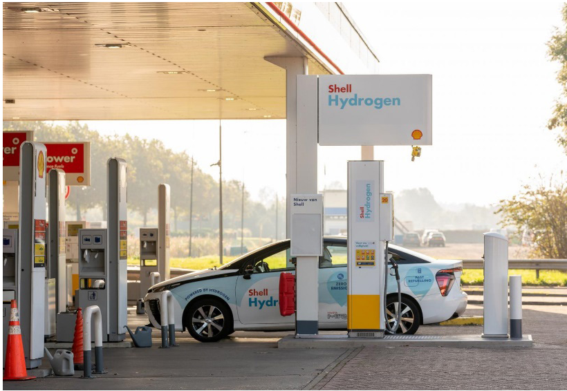
Figure 1. A hydrogen refueling station in the Netherlands by Shell 11
