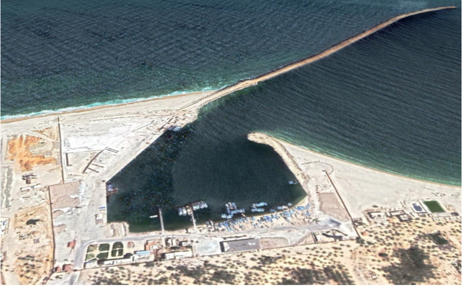
Figure 9: Aerial photo of the Port of el-Arish 21
