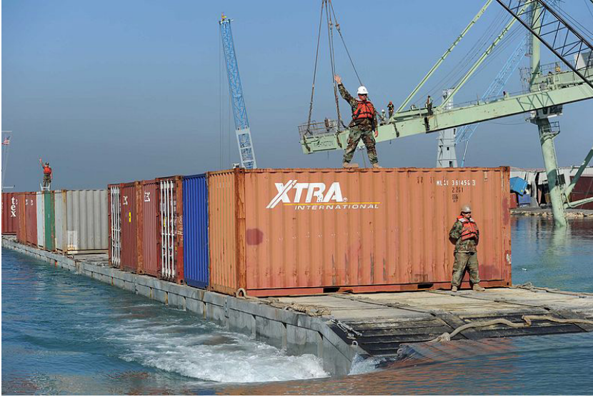
Figure 7: A floating pier
