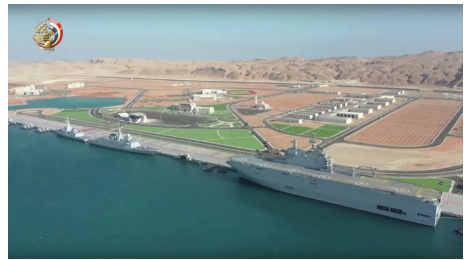
Figure 16: The new port in Ras-Banas
