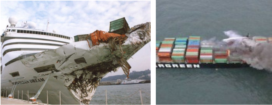
Figure 9: Damage from collision of container ship Ever Decent and passenger ship Norwegian Dream in 1999
