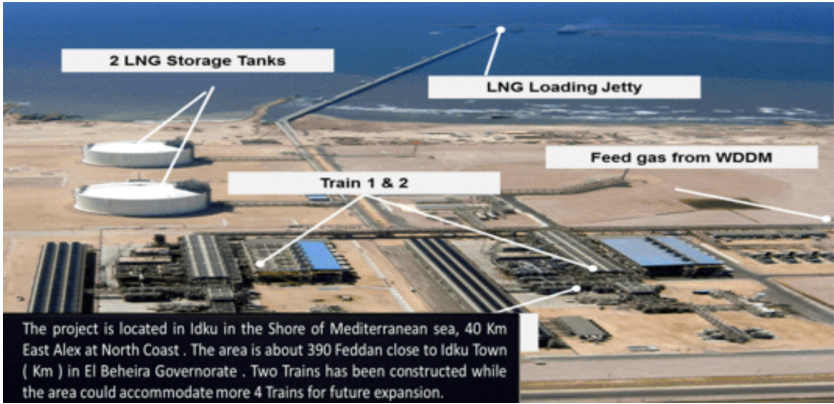
Figure 7: Idku LNG plant with an annual production capacity of 7.2 million tons of liquefied gas and the potential for a further increase 36
