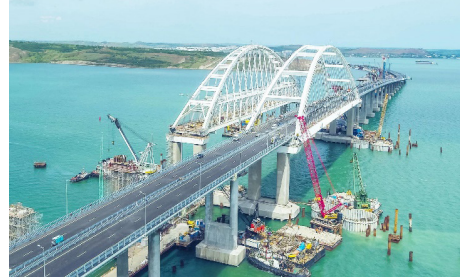
Fig. 4: The Crimea Bridge under construction
