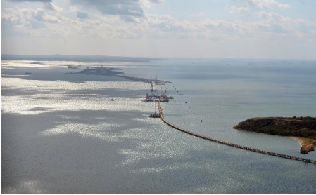
Fig. 5: Construction of the bridge over the Kerch Strait
