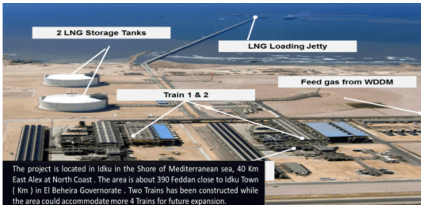
Figure 7: Idku LNG plant with an annual production capacity of 7.2 million tons of liquefied gas and the potential for a further increase 36
