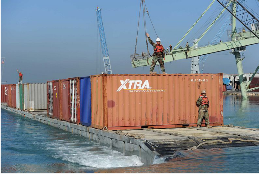
Figure 7: A floating pier
