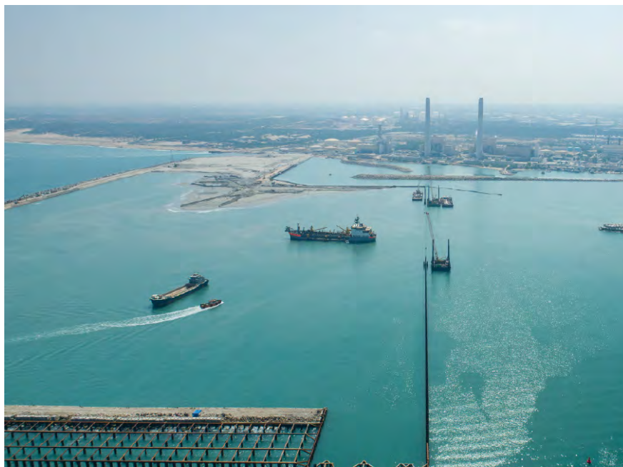
Figure 7 – The drained area of the Hadarom port (as of mid-2017)
