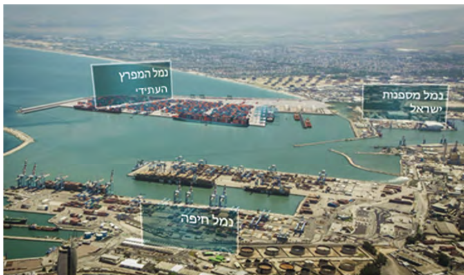
Figure 1 – The Hamifratz port will be built next to the Port of Haifa and the Israel Shipyards port.
