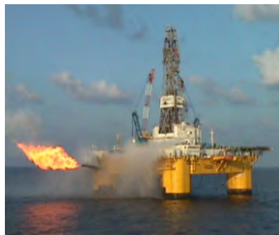
Figure 12 – Drilling rig ("Marine Installation")
