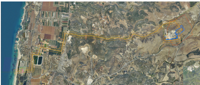
Figure 2: The condensate pipeline route from the Dor Valve Station ("DVS") to the "Hagit" site
