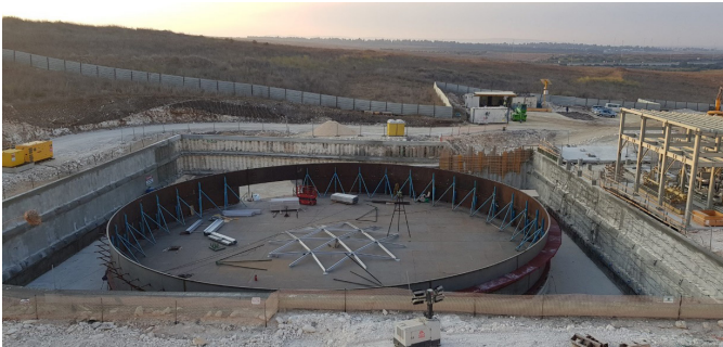
Figure 3: Construction of the Condensate Tank at Hagit for the Leviathan Project 9
