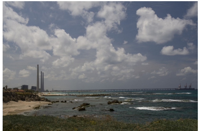
Figure 4: The Orot Rabin Power Plant as a preferred location for the construction of a Condensate Farm for export purposes
