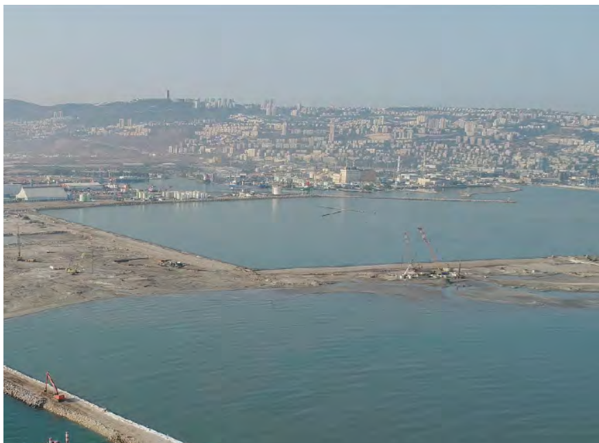
Figure 4 – The extension of the Port of Haifa breakwater and the drained area of the Hamifratz port (as of mid-2017).
